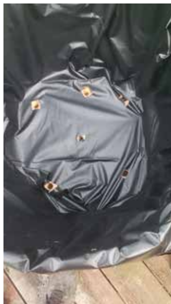
Top Left: Several one-inch drainage holes were drilled into the bottom of each planter. The holes needed to be covered to hold the dirt in place. Using some leftover copper screen from the windows of the house (stronger than fiberglass and will last my lifetime), I stapled the copper screen into place.
