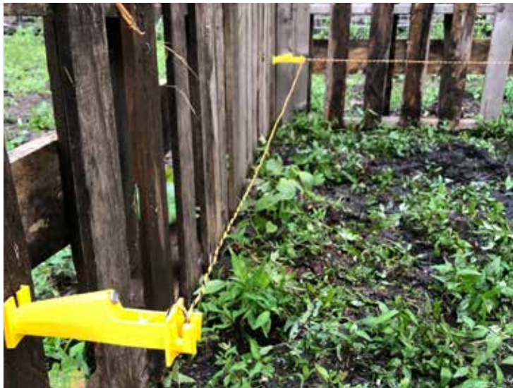
Install the electric wire between six inches and 12 inches above ground level.
